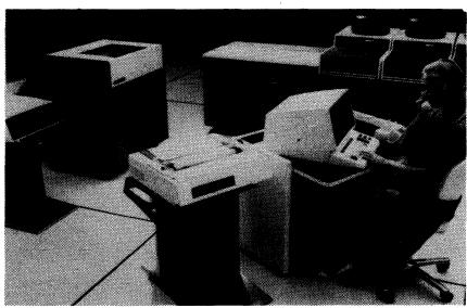
A typical small DPS 7 configuration includes the operator console and printer plus (left to right) a diskette drive, high-speed line printer, the DPS 7/35 central processor, and three disk drives. The DPS 7 has from one to four megabytes of memory, and supports a wide variety of peripheral devices.
