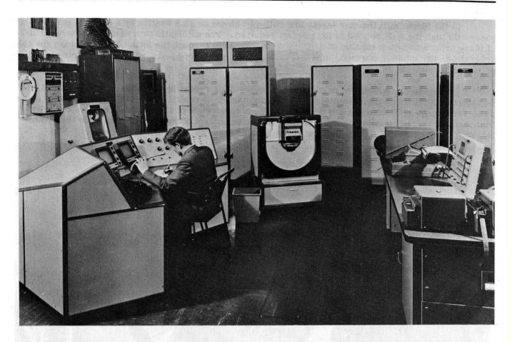
PRODUCTION CONTROL CENTER AT PARK GATE. THE OPERATOR CAN GIVE INSTRUCTIONS TO THE COMPUTER OR TALK TO MILL CREWS THROUGH MICROPHONE.
